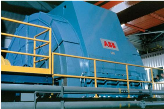
*New 100-MW (135,000-HP) synchronous motor used to operate the NTF wind tunnel*
